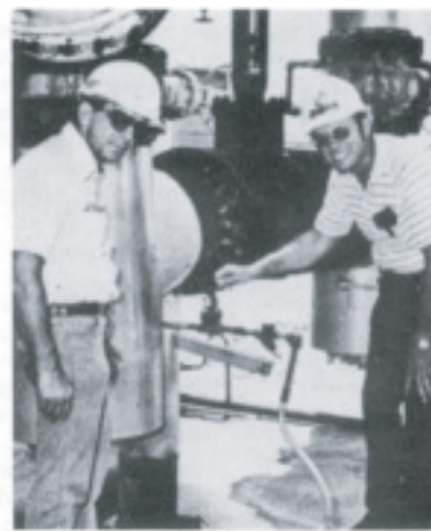
Peiper (right) and Bobby King, Swift Creek Maintenance Supervisor, review installation of Eagle Zero Steam Leak bellows valve
